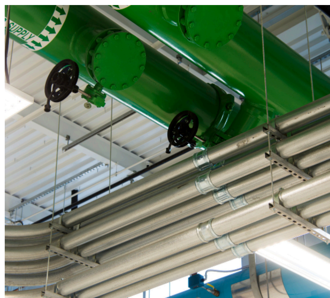
Mechanical, Electrical & Plumbing Services (MEP)
