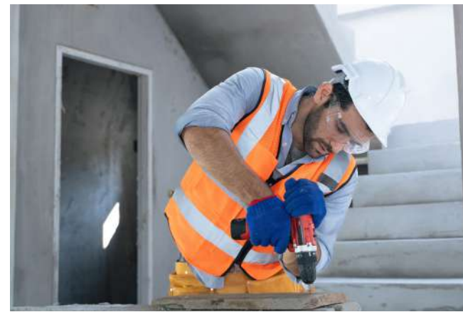
Construction tools & PPE
